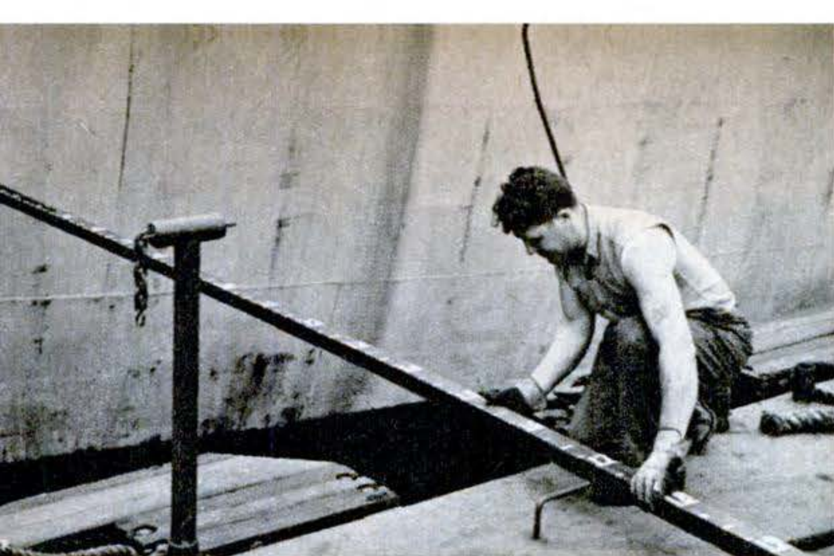
3. Measurements with this giant "ruler" help center vessel in dock. After she reaches correct fore-and-aft position, men on dock use power capstans and block-and-tackle rig to move her sideward until she is lined up over the blocks that will support her keel.
